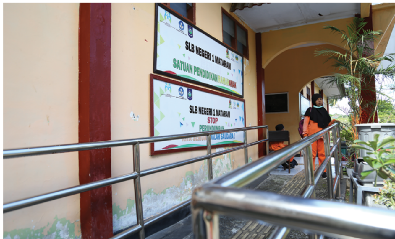
Soleha's school are equipped with holder bar to make it easier for students who have walking difficulties or unable to see. (Photo: Plan Indonesia)
