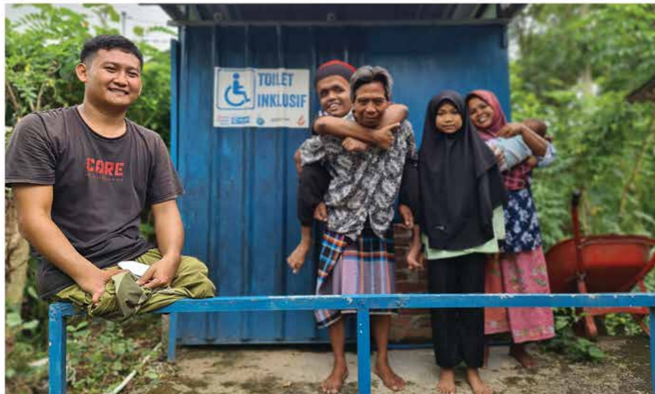
In Lombok Tengah District, the Wusan Pade Angen Group has also constructed several disability-friendly latrines that can mitigate the risk of accidents for users. (Photo: Musfarayani/Doc. Plan Indonesia)
