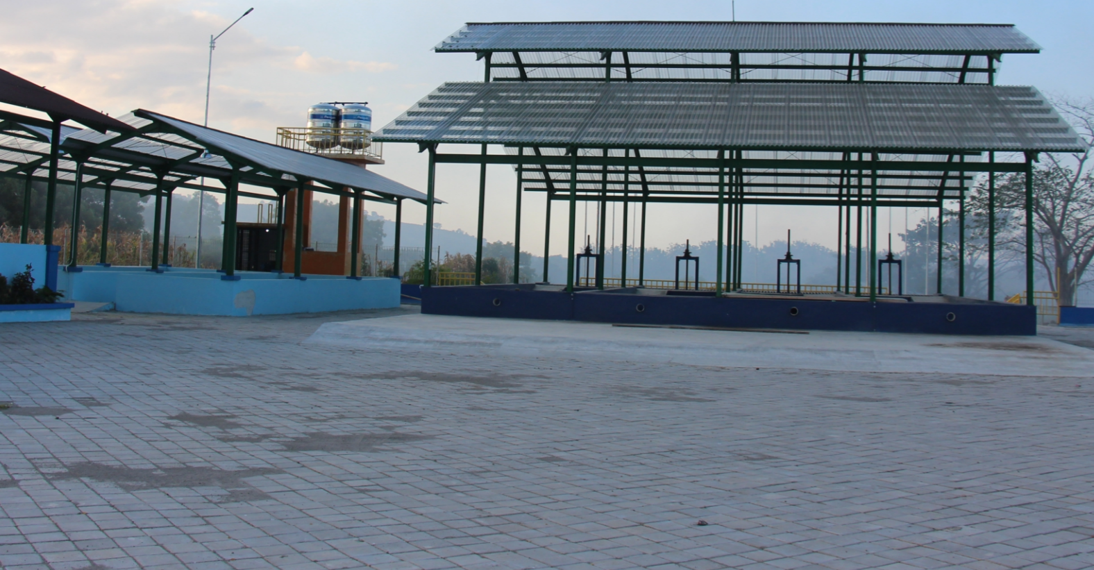
Solid Separation Chamber (SSC) and Sludge Drying Bed (SDB) in Raberas FSTP Sumbawa. The sludge which settles in the Solid Separation Chamber is manually drawn and dried out in Sludge Drying Bed.
